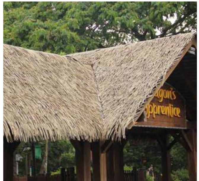
The finished look
